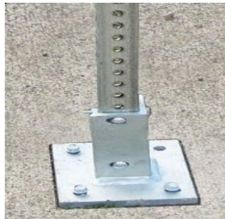
Figure #47: Sign being mounted into the concrete
