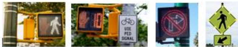
Figure #8: Examples of Various Signalized MUTCD Compliant Signs
